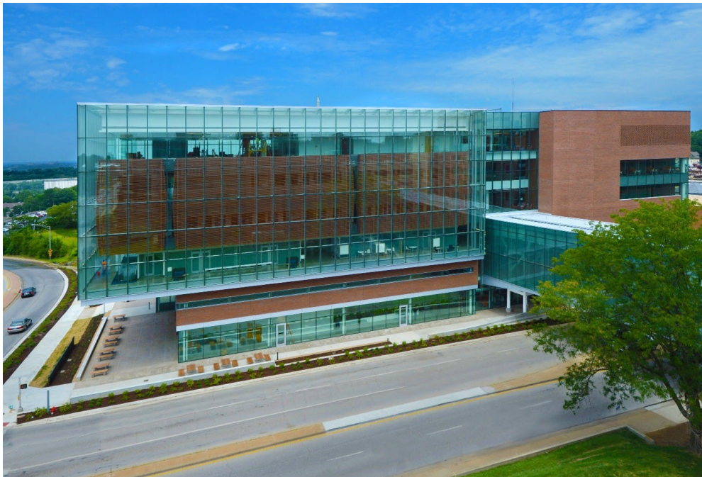
Health Education Building at the University of Kansas Medical Center, viewed from the south.
